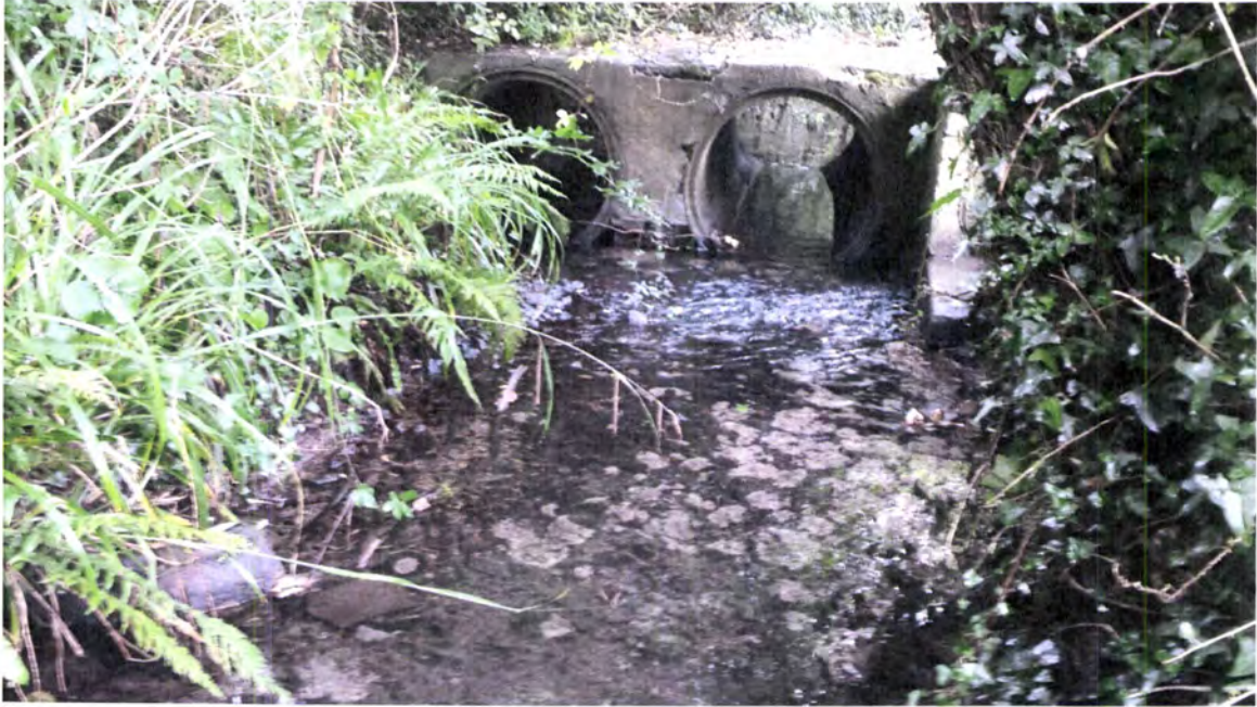
Culvert within the site to be removed.
